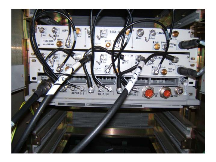
Nortel Networks MFRM3 Assembly Front View Fan Assembly Removed
