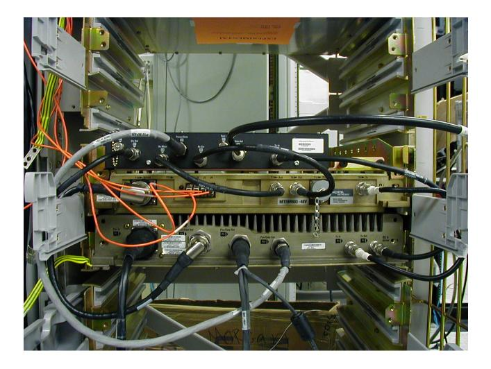
Nortel Networks MFRM Assembly Front View Fan Assembly Removed
