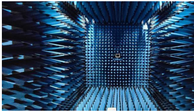
Figure 2: Geometry of Anechoic Chamber for Radiation patterns.
