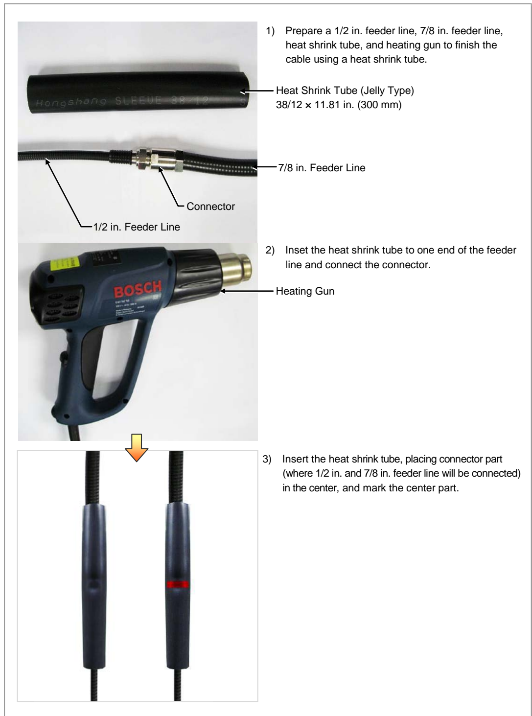
Figure C.17 Shrinking the Heat Shrink Tube-Connector (1)
