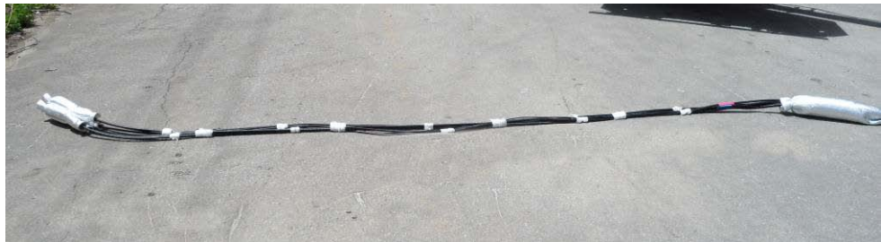
Figure 2.19 Installing Hybrid cable (2)
