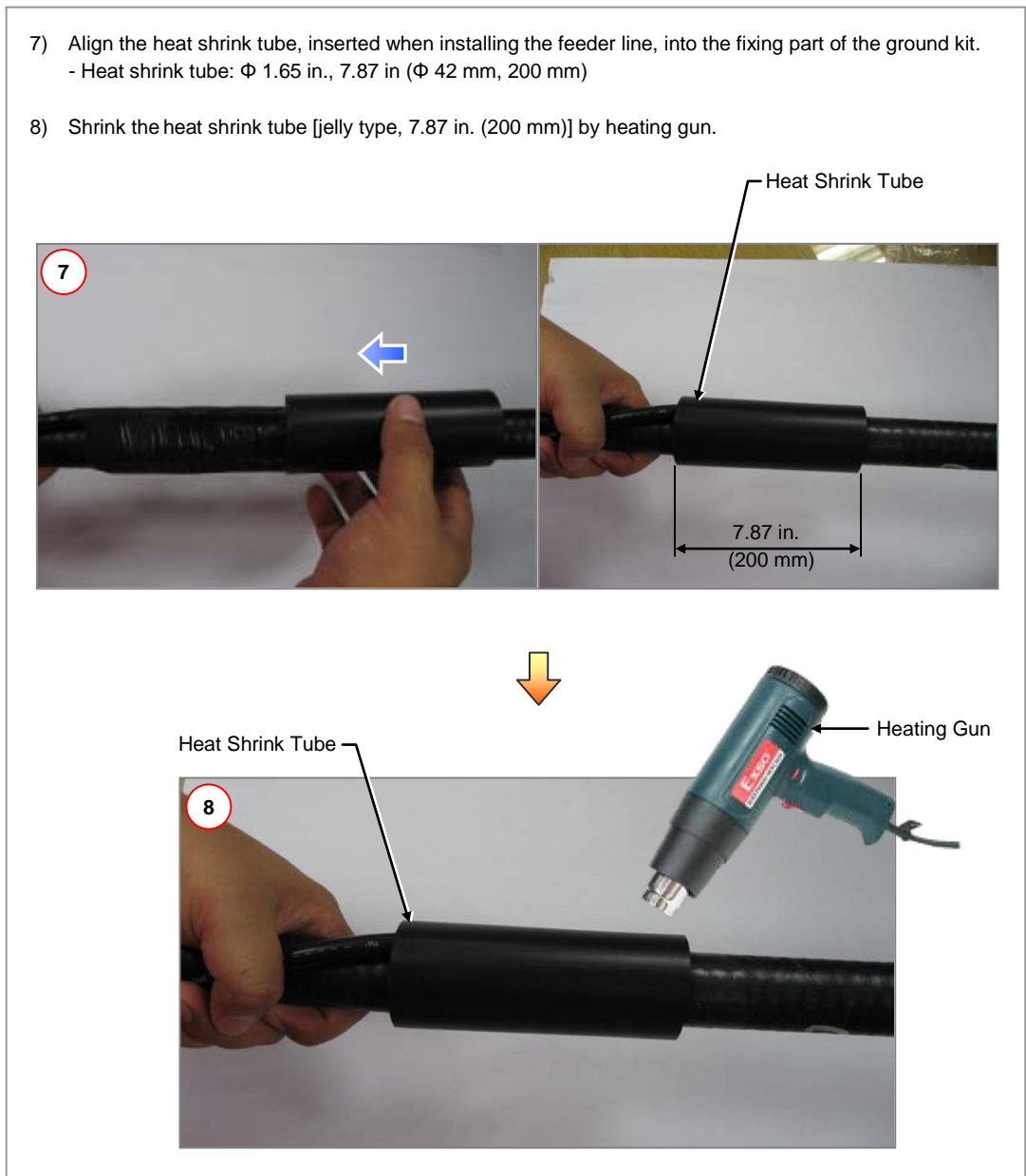
Figure B.3 Feeder Cable Grounding (3)
