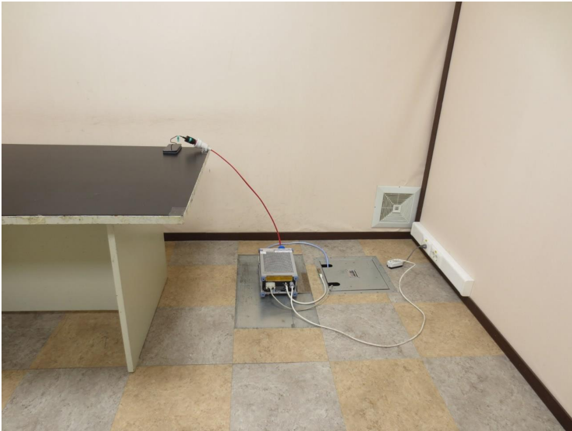
Position: Aligned, [25 W]
