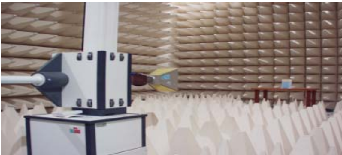
Figure2. Photograph of 3m Fully Anechoic Chamber
