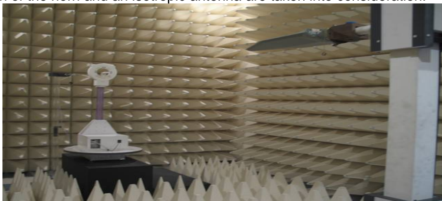
Figure2. Photograph of 3m Fully-Anechoic Chamber
