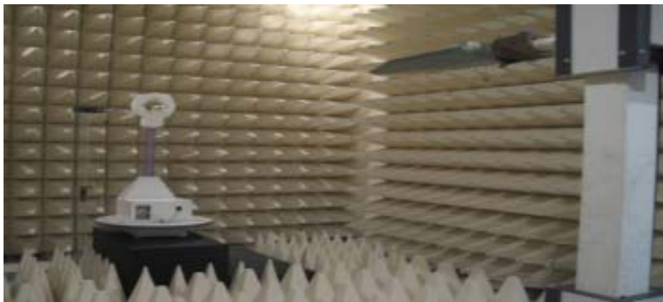
Figure2. Photograph of 3m Fully-Anechoic Chamber
