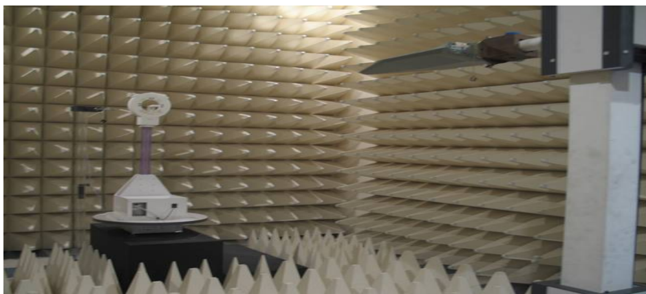
Figure2. Photograph of 3m Fully-Anechoic Chamber
