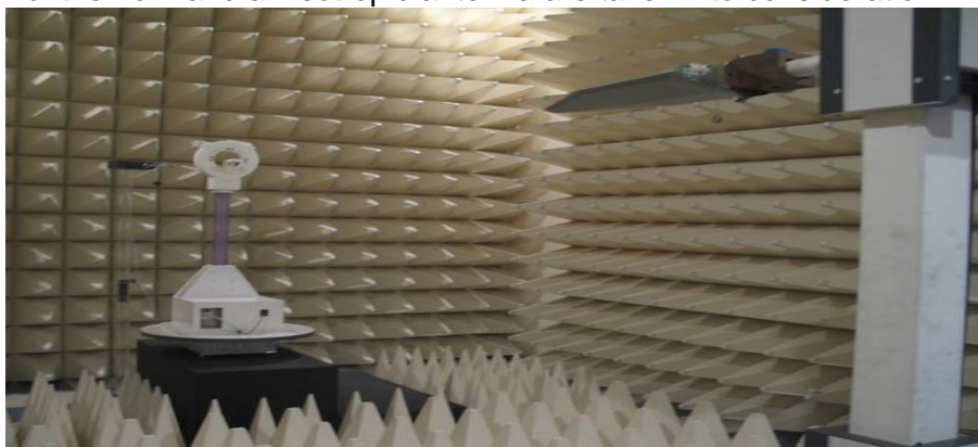
Figure2. Photograph of 3m Fully-Anechoic Chamber
