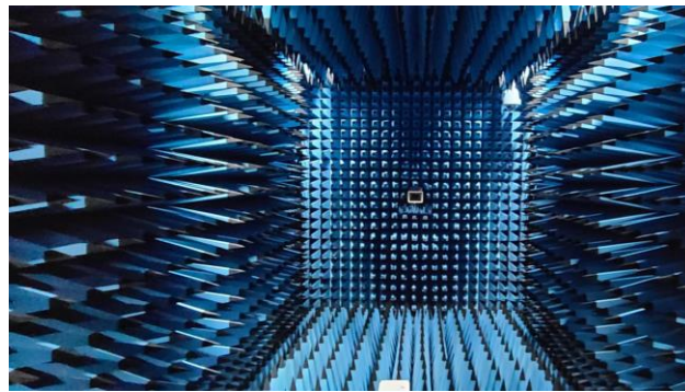
Figure 2: Geometry of Anechoic Chamber for Radiation patterns.
