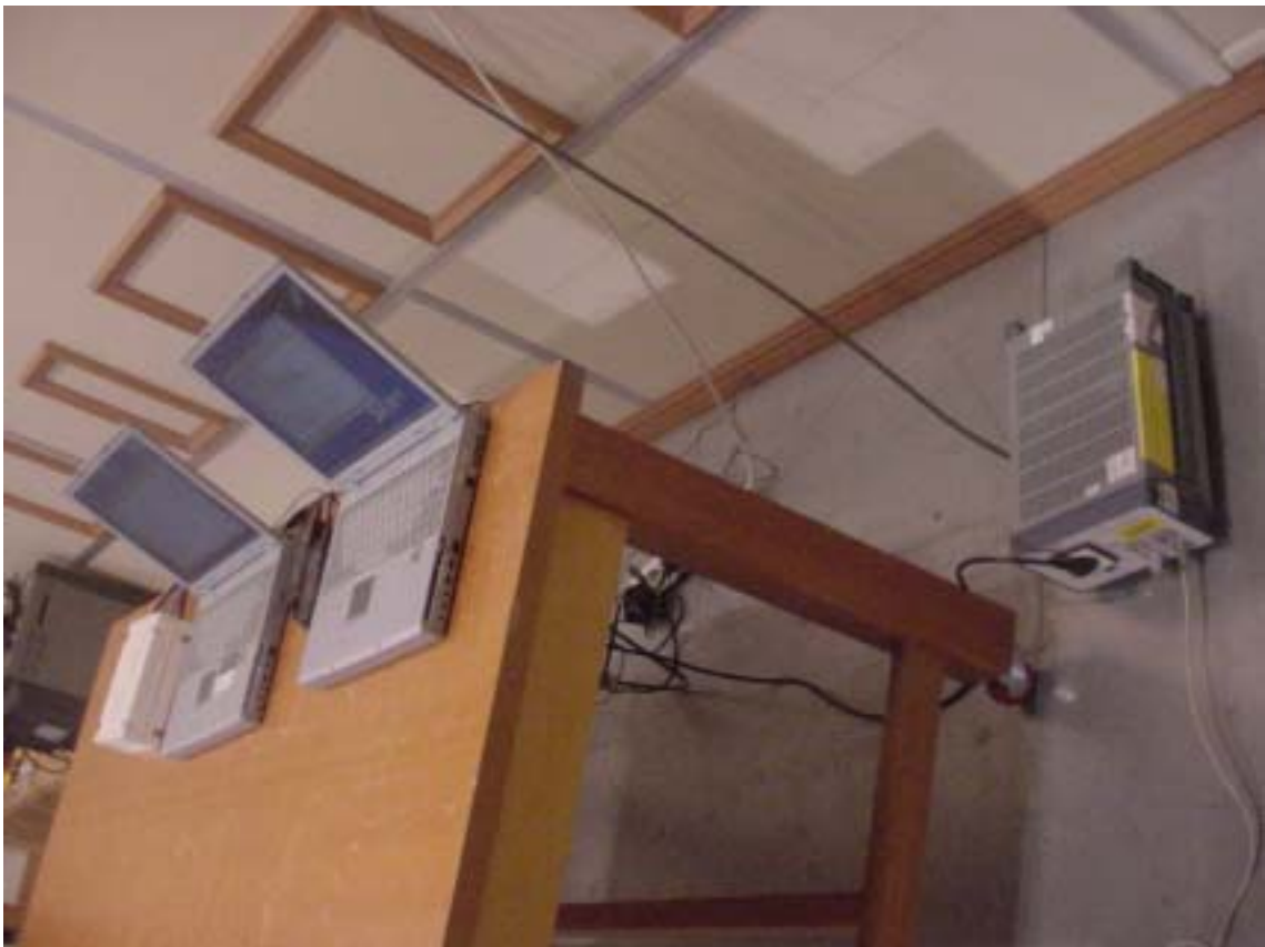
<SIDE PHOTO OF CONTINUOUS DISTURBANCE VOLTAGE >
