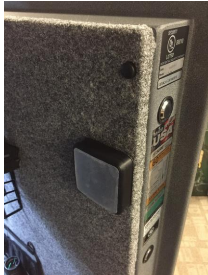
Magnet is mounted on side wall of vault to align with the Puck
