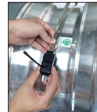
② Put the sensor on the steel tie
