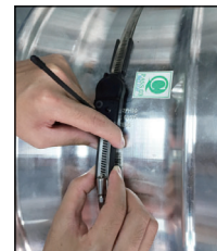
④ Installing non-slip rubber pad
