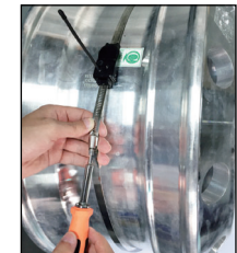
③ Pre tighten steel tie screw
