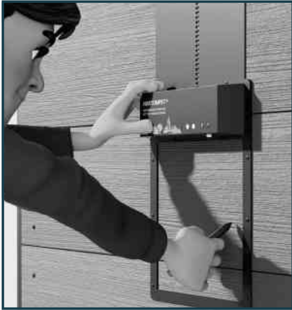
1. Mark the location of the opening on a flat surface.
