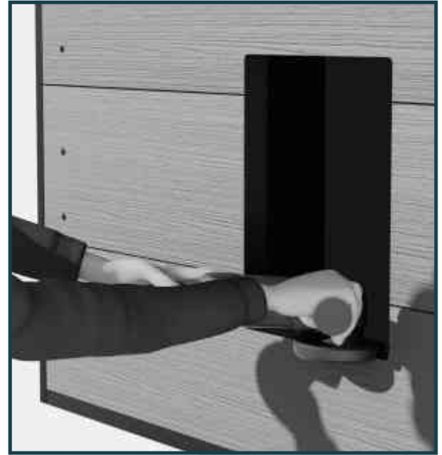
3. Saw off the opening by connecting the holes.
