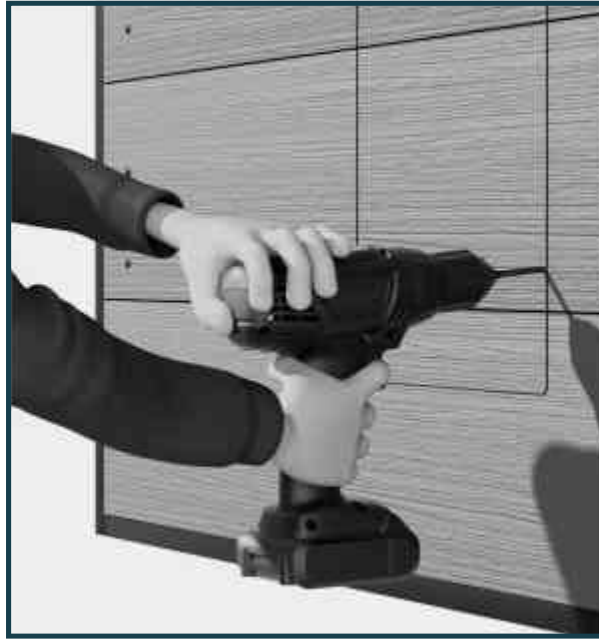
2. Drill at the corners of the marked opening.
