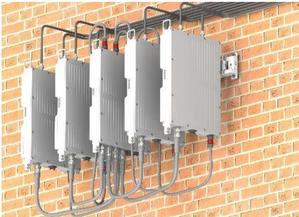
Figure 4-31 Connection for power between MCU and LPAs on the bottom
