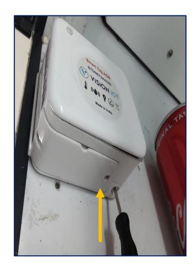
Tighten the backplate screw using the screwdriver.
