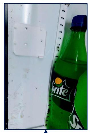
Measure the Position to Fix the Smart device and Stick the Back Plate Using a Flat Head Screw into the Cooler.
