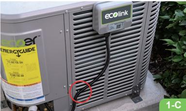
02. Unscrew the cable locker cap and securely fasten the waterproof joint to the reserved hole (plug has to be removed).
