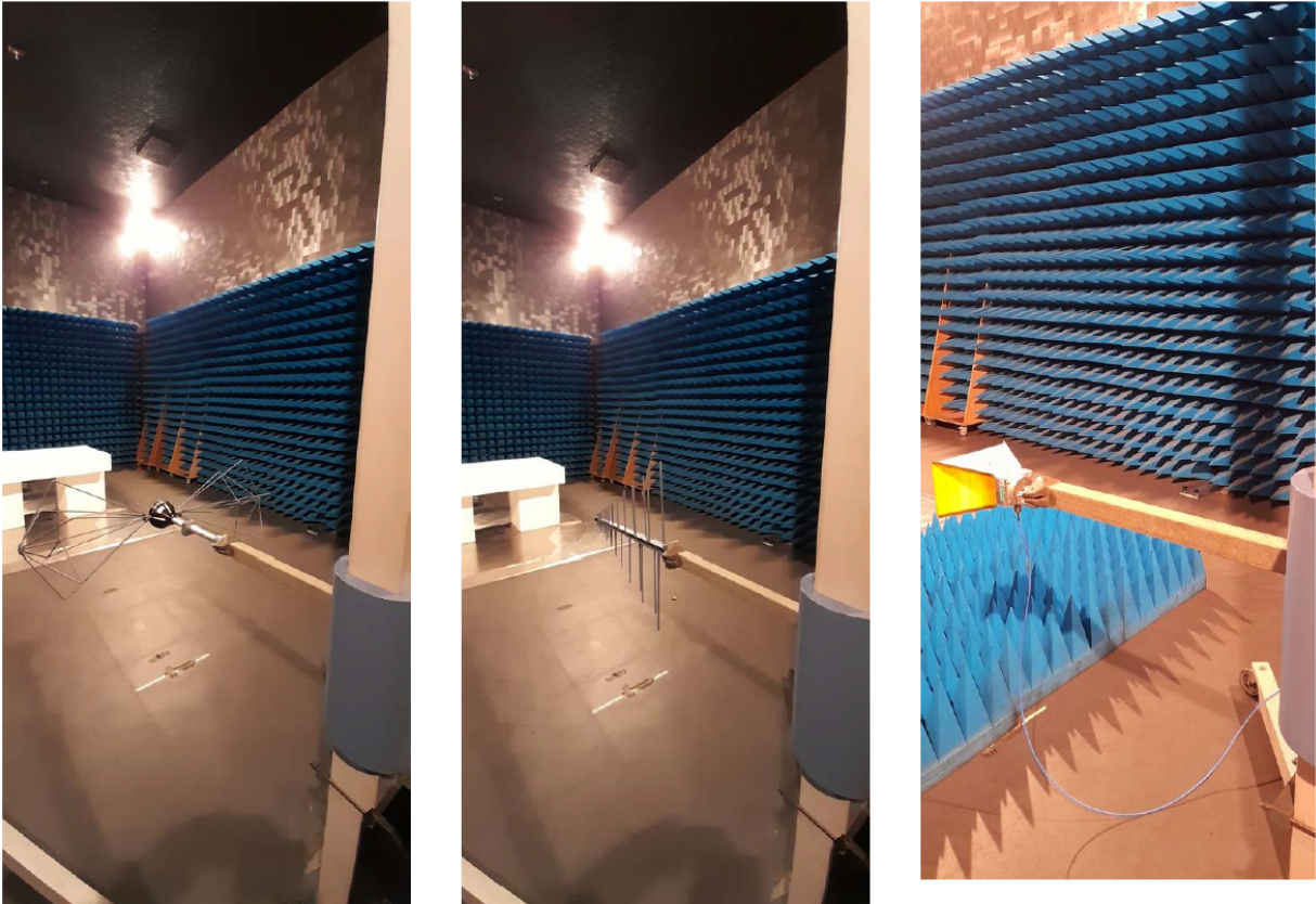
Photo antenna tower :
