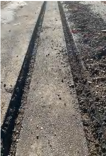
Asphalt Cut Total 23cm/9in depth
