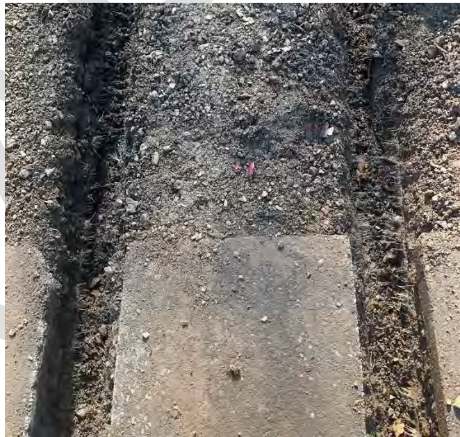
Asphalt to Soil transition maintain 23cm/9in depth
