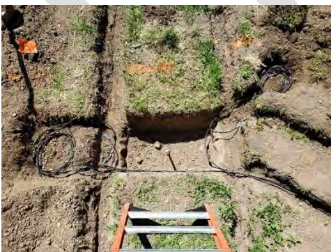
Sensor cables and lead-in cables in place
