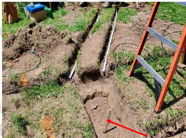
Install Ground Rod in between the DM's
