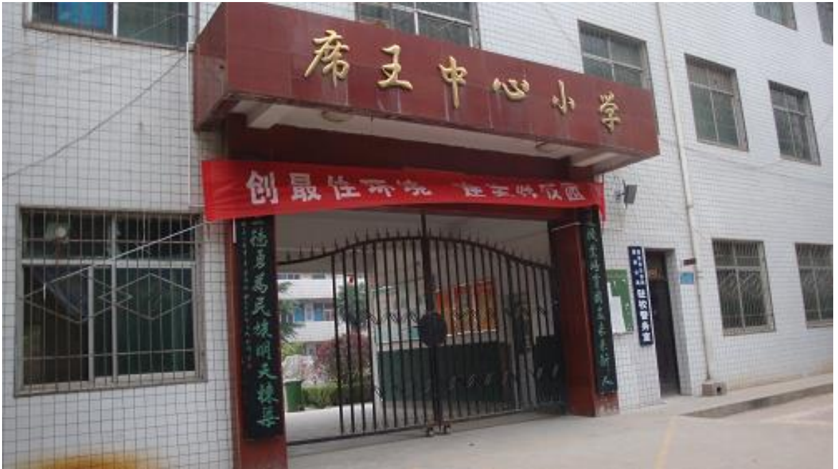
Figure 6-1: Install JAVS18-9003B new generation campus access management system at the school gate
