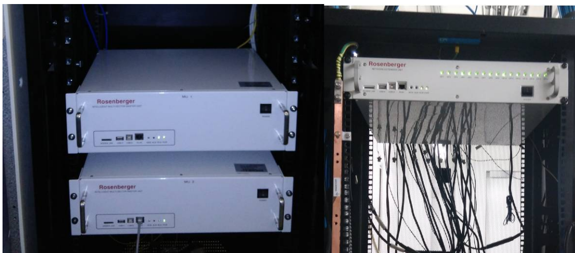
Figure 17 Installation of IM2U and NEU
