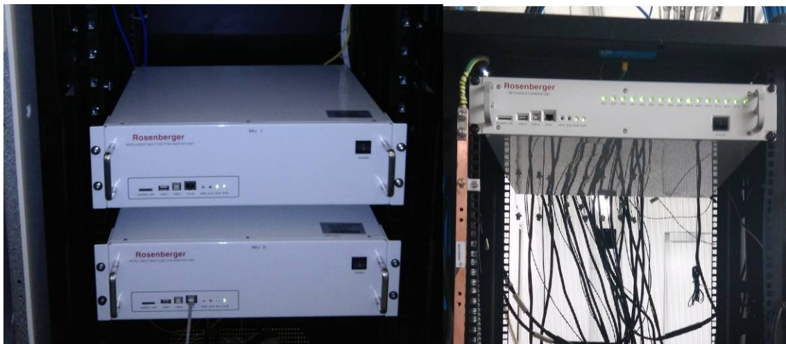
Figure 17 Installation of IM2U and NEU
