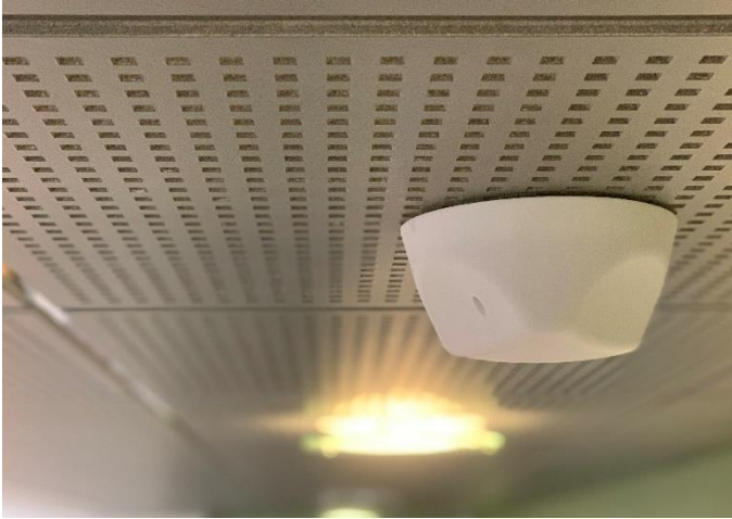
Figure 6 Example of beacon 3 mounting plate installation.
