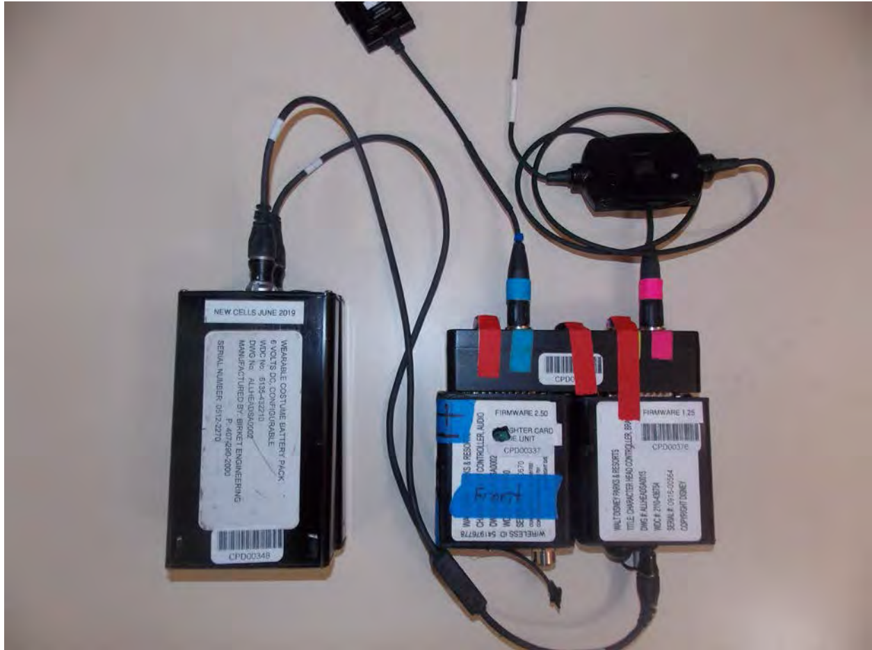
Unit Showing all Cabling
