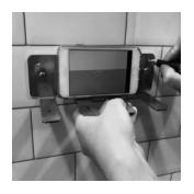
4. Hold the bracket to the desired location, using a level to confirm the bracket is straight. Mark the 4 mounting holes on the wall.
