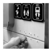
6. Take the anchors and press them into each hole until the anchor's lip is level with the wall.
