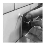
7. Place a screw through each of the wall-facing holes on the mounting bracket. Align the screws to the anchors on the wall.
