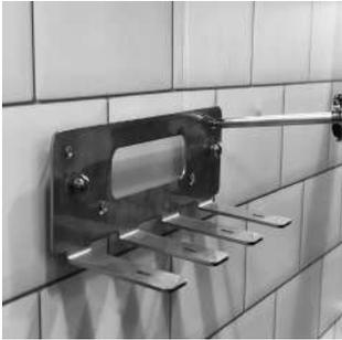
8. Use your screwdriver to mount the bracket to the wall by tightening the screws into the anchors.
