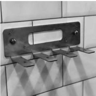
9. Tighten each screw so that the bracket is flush with the wall.
