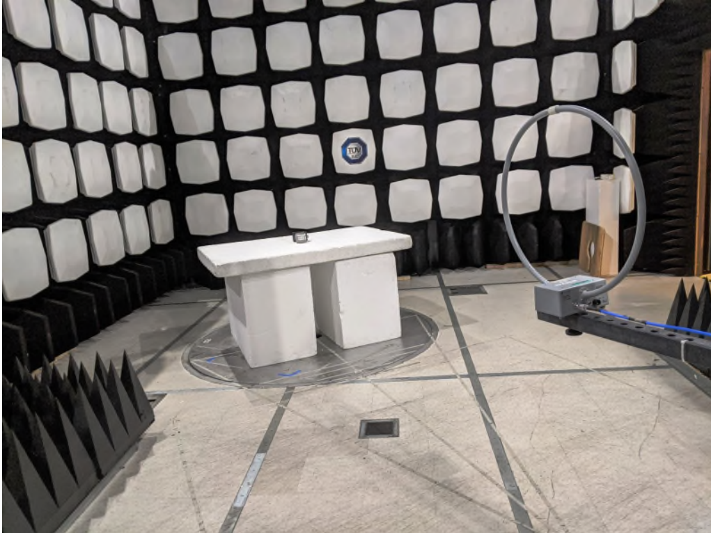
Figure 2: Equipment Under Test – Radiated Emissions <30MHz
