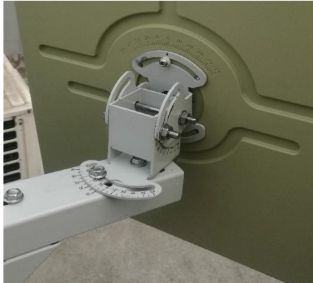
Figure 5-1-2-1 Bracket fixed of antenna body
