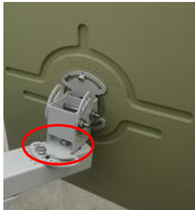
Figure 5-3-3-2 Azimuth adjustment diagram
