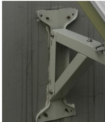
Figure 5-1-2-2 Schematic diagram of expansion screw fixation
