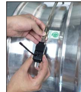
② Put the sensor on the steel tie
