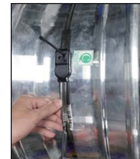
⑤ Tighten the steel tie screw
