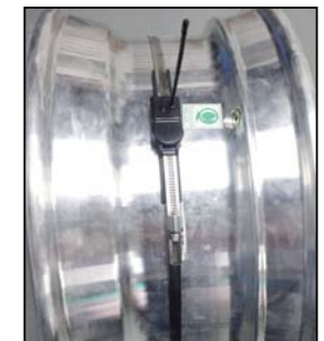
⑥ Installation Completed
