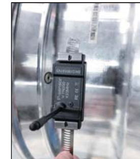
②Put the sensor on the steel tie
