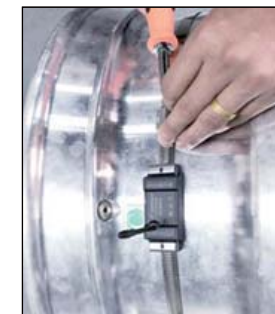
⑤Tighten the steel tie screw
