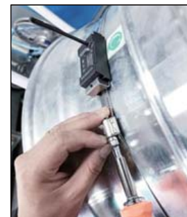
④nstalling non-slip rubber pad
