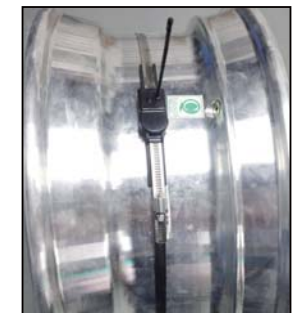
⑥ Installation Completed
