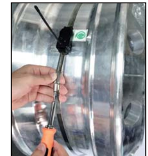
③ Pre tighten steel tie screw
