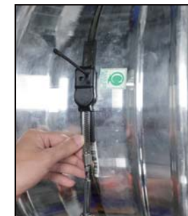
⑤ Tighten the steel tie screw
