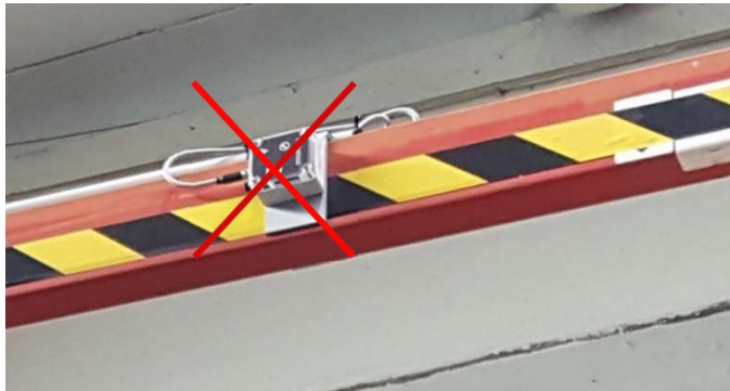
Example of how it shouldn't be done: horizontally mounted on metal sheet
