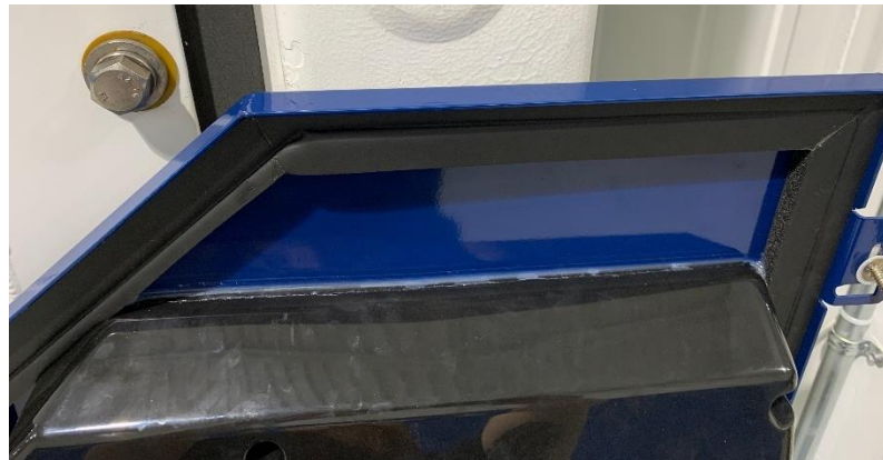
Figure 7b: Caulking of Rain Shield
