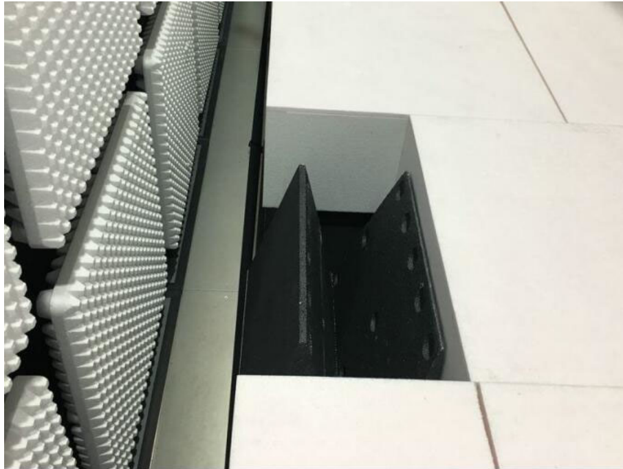
There are absorbing materials under the ground
