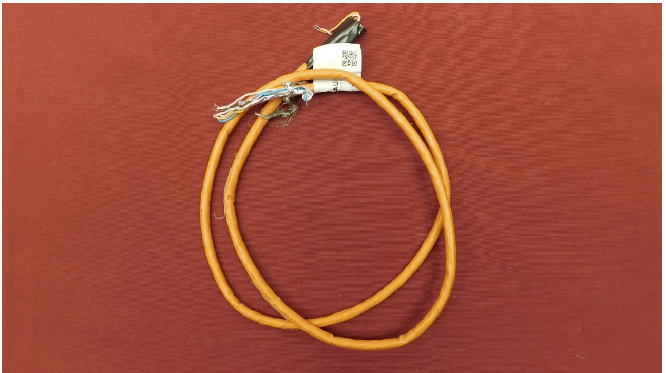
Picture 8: Used cable
