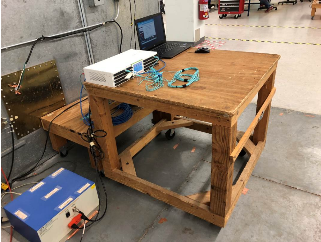
Two Power Supplies
