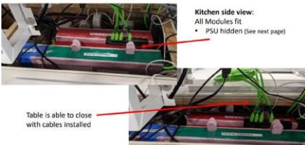
All Module installed on Brackets
