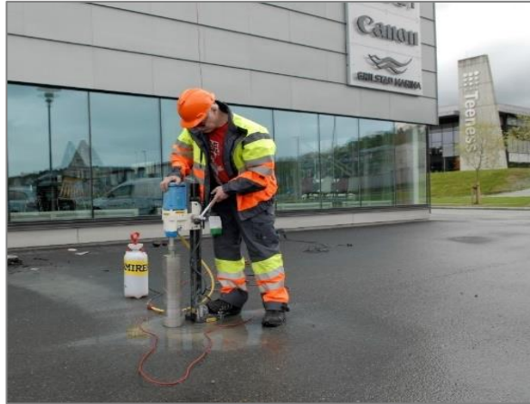
Picture 3 Coring the sensor hole
