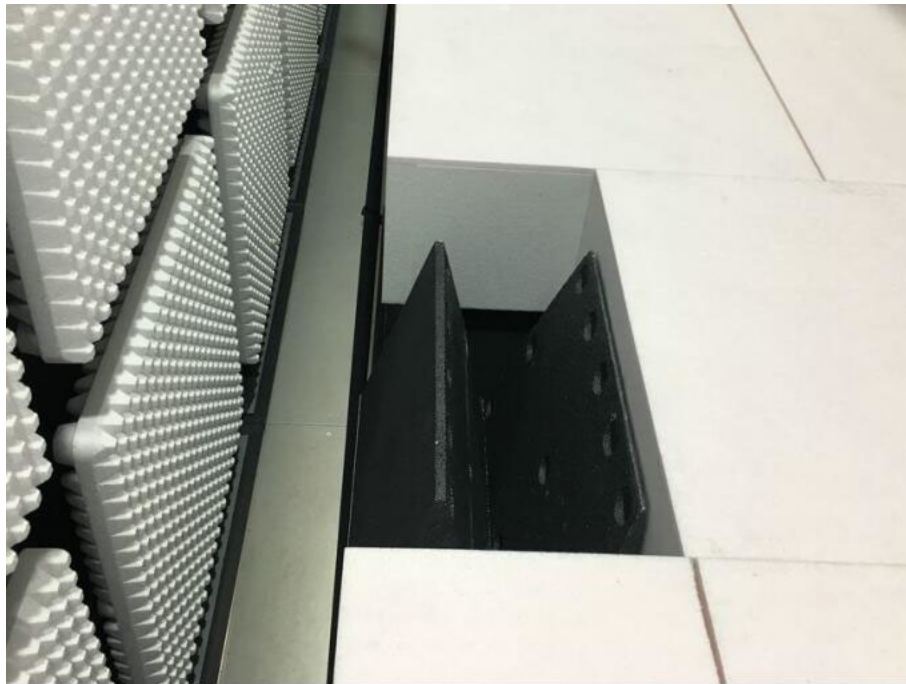
There are absorbing materials under the ground
