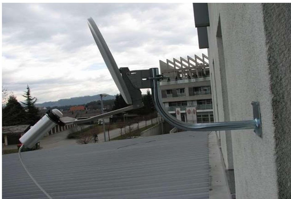
Figure 4. CASE1: suitable antenna site installation
