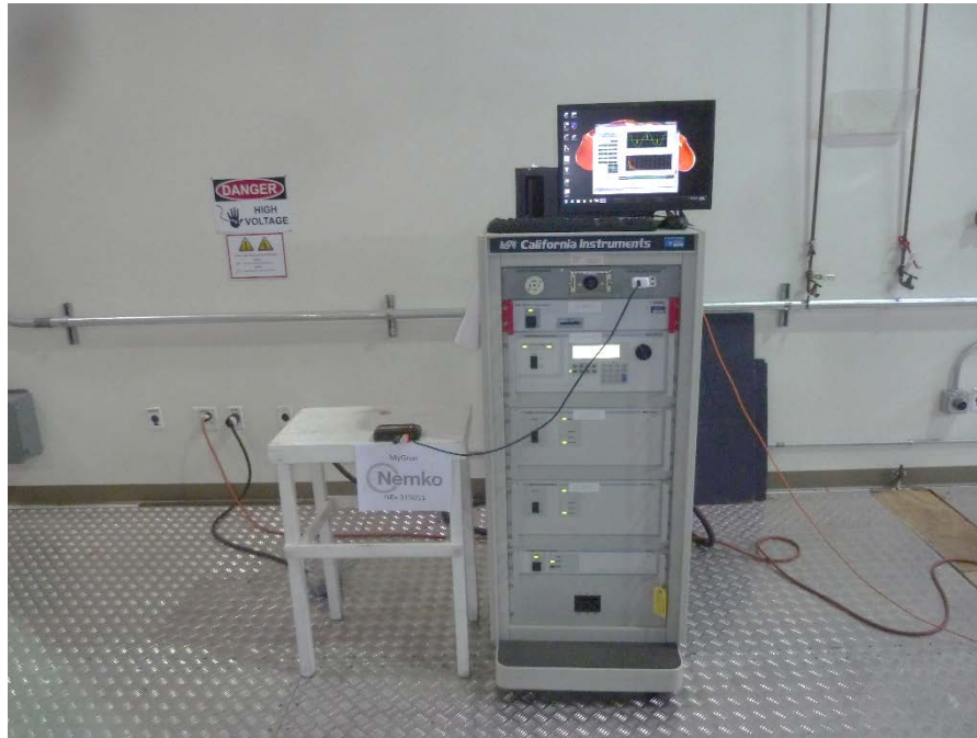
Figure 8.3-1: Clause 8.6 – Voltage fluctuations and flicker (AC mains input port) setup photo
