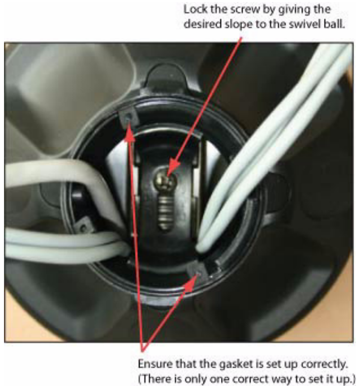
Figure 17 Routing the cables into the swivel
