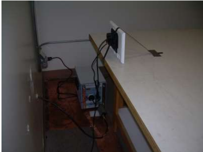
Photograph 11 – Back View Conducted Emissions Configuration – In-wall Units AC Powered
