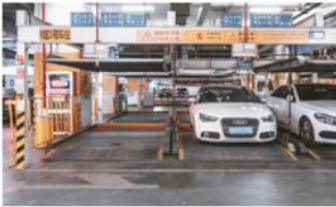
Parking lot Management
