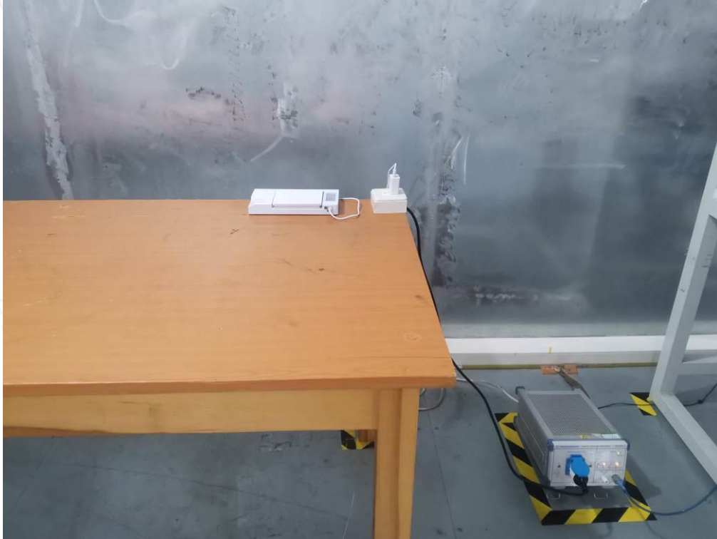
Photo of Power Line Conducted Measurement
