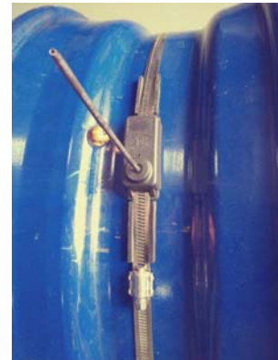
4、 Installing non-slip rubber pad 5、 Tighten the steel tie screw 6、 Installation completed
