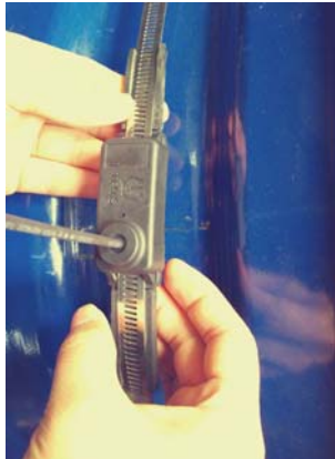
4、 Installing non-slip rubber pad 5、 Tighten the steel tie screw 6、 Installation completed
