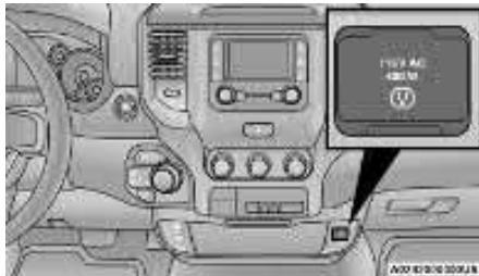
Center Stack Power Inverter
