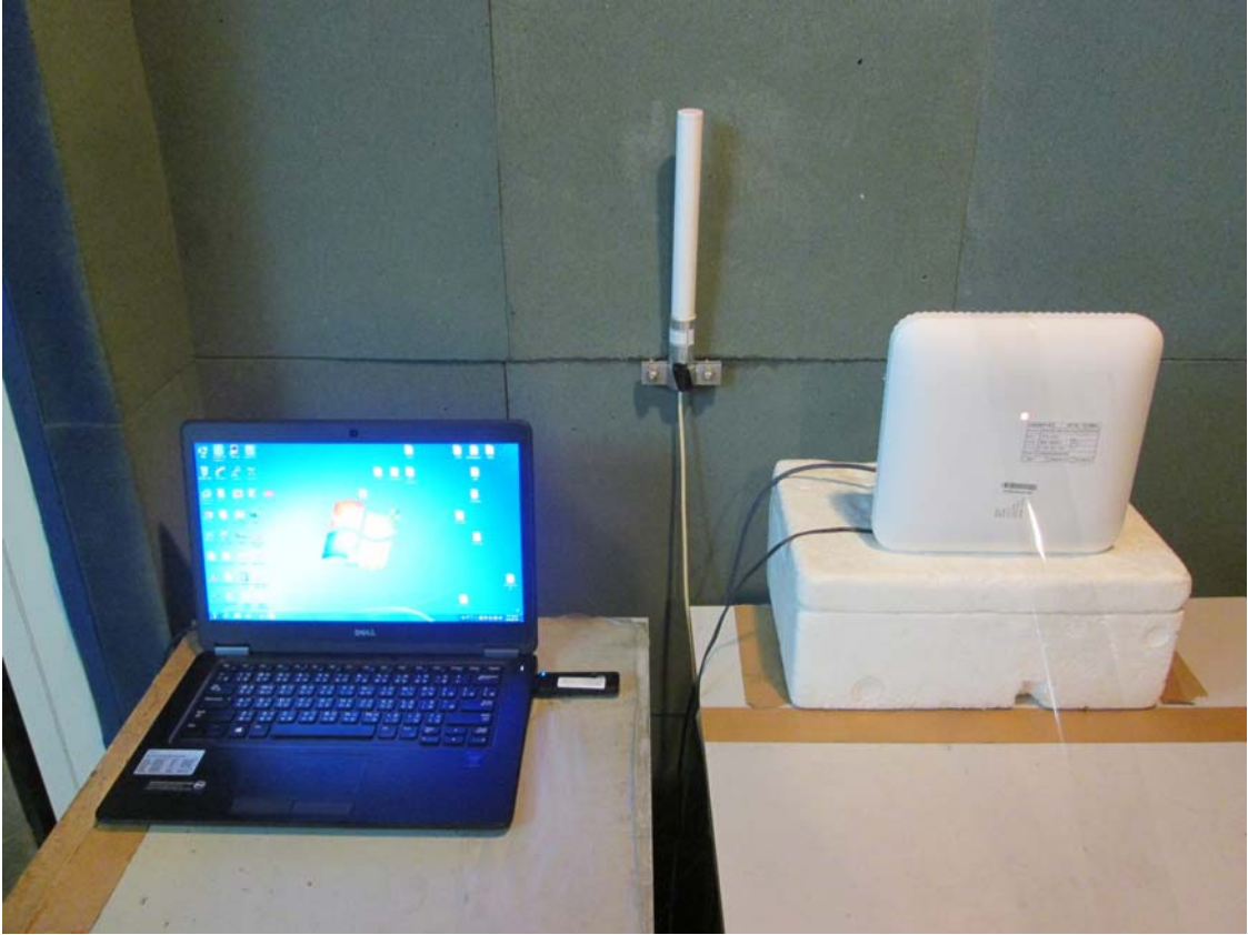
Test results demonstrating Master links with Client on a test frequency.
