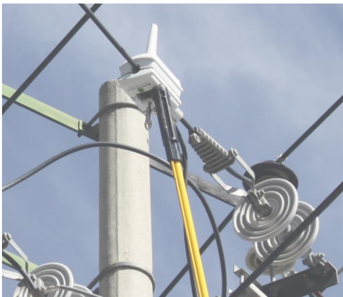
Figure 24: Fasten the secondary clamp screw
