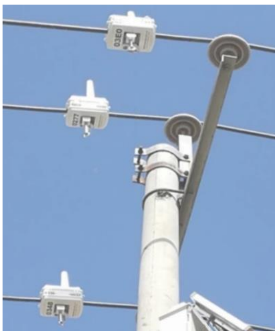
Figure 29: Sensor installed on each phase
