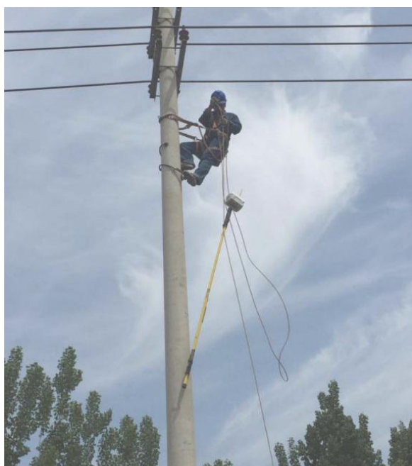
Figure 31: Lifting the equipment using a climbing equipment and a rope
