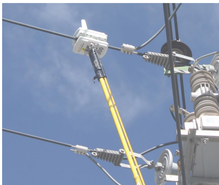
Figure 22: Fastening the main clamp screw
