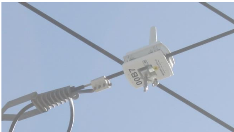
Figure 23: Sensor attached to wire but still open
