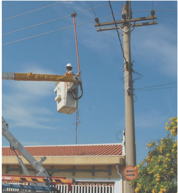
Figure 34: Installation by hot stick using a crane
