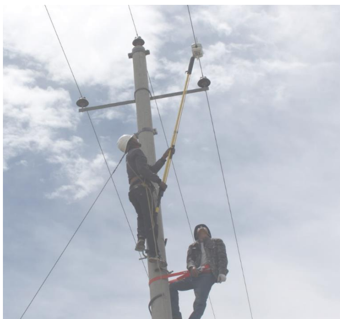
Figure 32: Installation by hot stick (fastening the secondary clamp screw)
