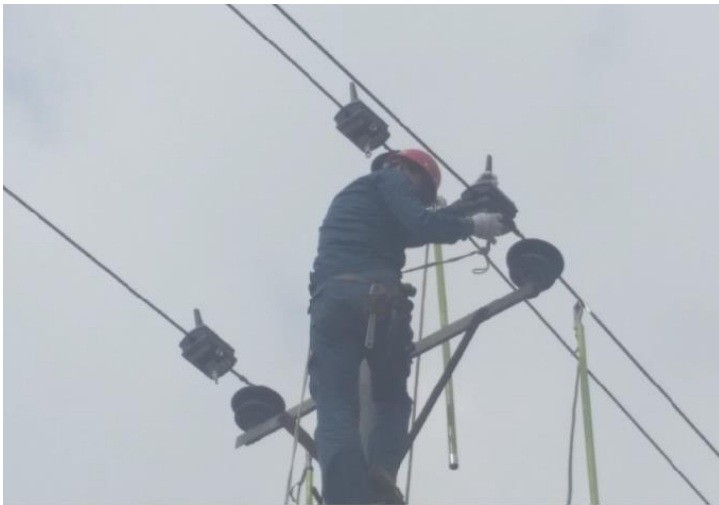
Figure 26: Direct installation on a non-energized line
